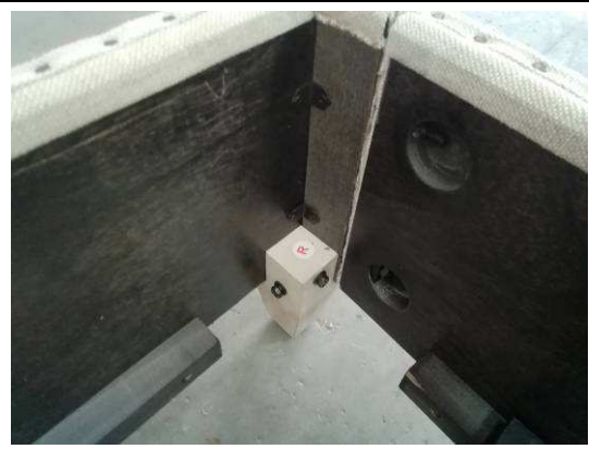
The close-up view of the construction
