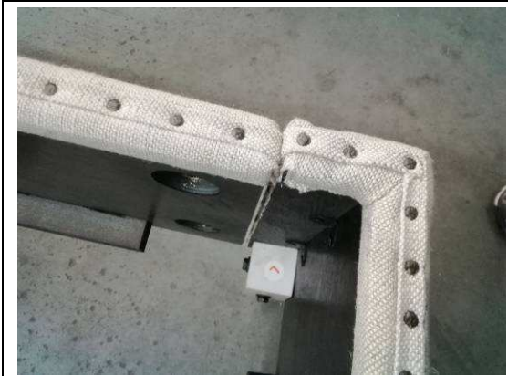
The close-up view of the construction
